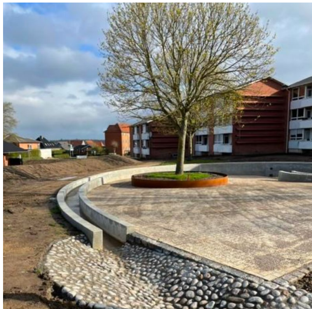
Nørgaard has conducted earthworks and construction work for Brændkjær Climate Park
